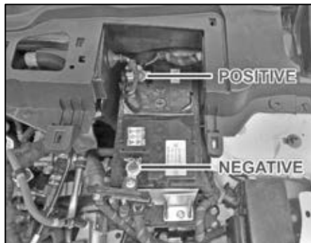
Battery location- Petrol
